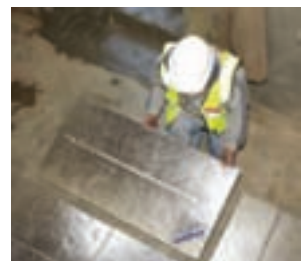
With an aged lambda of just 0.007W/m.K, VIPs can provide solutions for areas that would previously have remained un-insulated because space was an issue
