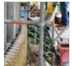
The natural stone ‘bricks’ laid in dogtooth alignment, giving a basket weave appearance
