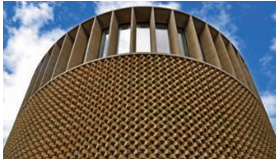
The natural stone ‘bricks’ laid in dogtooth alignment, giving a basket weave appearance
