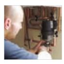
Sentinel's new technology heating system filter – Eliminator – has been very well received by installers all across the UK. The Eliminator's four powerful hydro-cyclones force clean water out of the top of the filter and spin all types of suspended system debris down into the bottom of the collection chamber. Four strategically positioned magnets accelerate the capture and removal of any magnetic debris. Vitally, the
