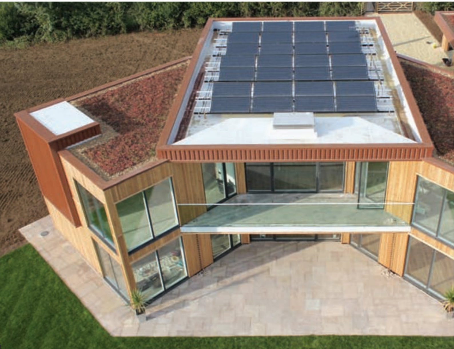
AERIAL VIEW OF THE HOUSE SHOWING SOLAR PV-T PANELS AND SEDUM GREEN ROOF (ABOVE) AND ILLUSTRATION OF THE WORKINGS OF THE SOLAR HOUSE (BELOW)
