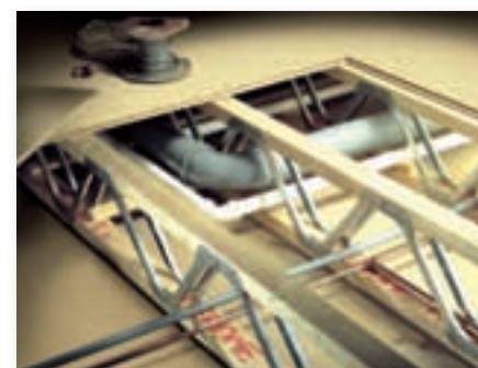
SECTION SHOWING TRUSSED RAFTERS IN PLACE AND SERVICES RUNNING THROUGH THE METAL WEB JOISTS © MITEK INDUSTRIES
