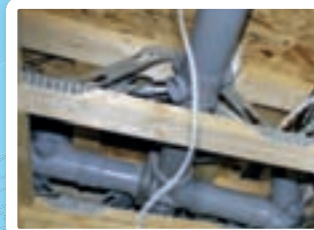
SpaceJoists easily accommodate services
