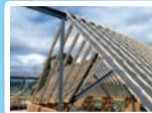
SpaceRafters provide large insulated roof spaces
