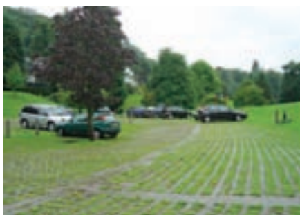
Above & right shows finished grass reinforcement
