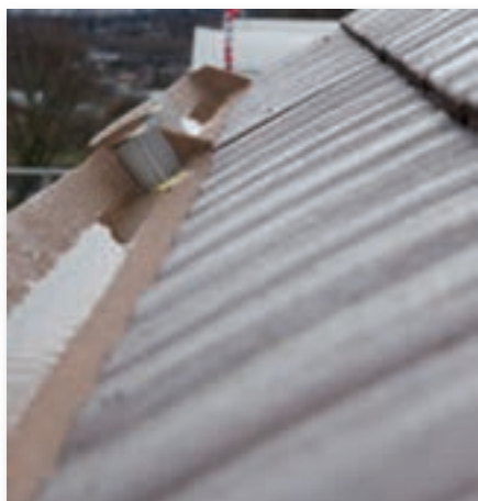
THIS RAINWATER HARVESTING SYSTEM USES RAINWATER COLLECTORS PLACED ACROSS THE WIDTH OF THE ROOF AND INTEGRATED WITH THE TILES. EACH COLLECTOR FEATURES A SELF-CLEANING FILTER THAT FILTERS THE RAINWATER BEFORE IT IS DIRECTED TO THE STORAGE TANK IN THE LOFT SPACE
