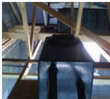
SOME RAINWATER HARVESTING SYSTEMS USE STORAGE TANKS PLACED IN THE EMPTY ROOF SPACES OF HOUSES TO ALLEVIATE PROBLEMS IN MAKING SPACE FOR AN ABOVE GROUND OR UNDER GROUND TANK
