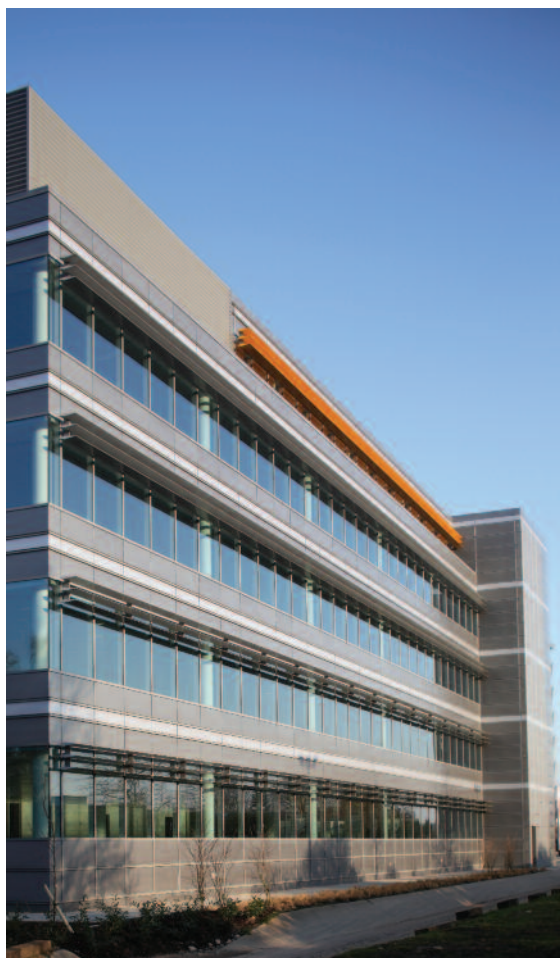
Horizontal fins (five groups of three fins), Velocity Building, Weybridge (right) and horizontal fins (two groups of six fins), University of Warwick, Mechanochemical Cell Biology Building (far right)
