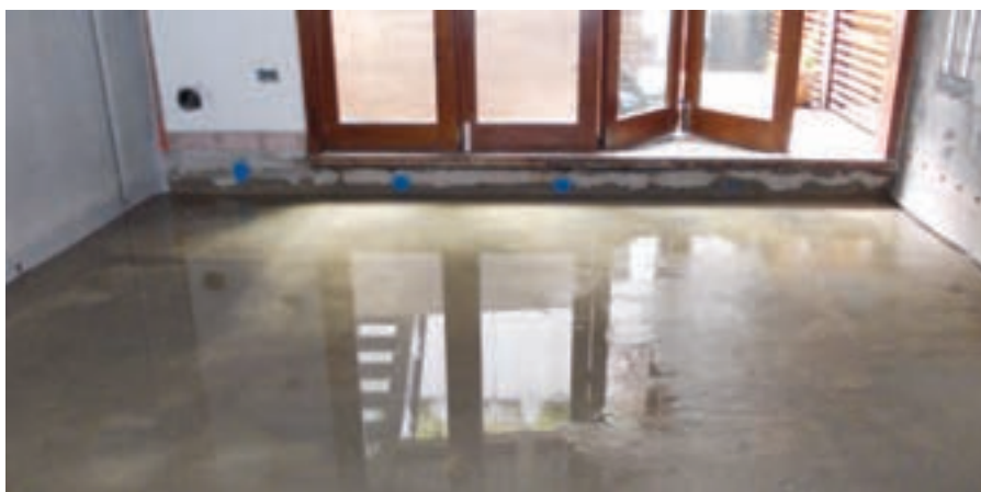
Example of basement waterproofing failure
