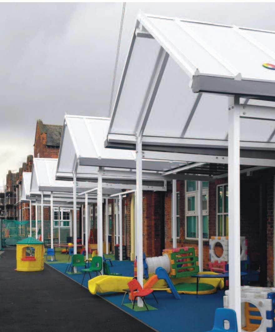
Above: Duo-pitched canopies glazed with panels fitted with multiwall polycarbonate – safe glazing for any school environment
