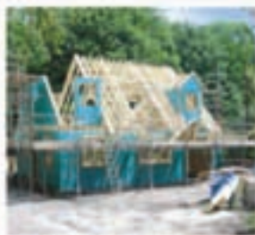
Watertight Frame Erection
