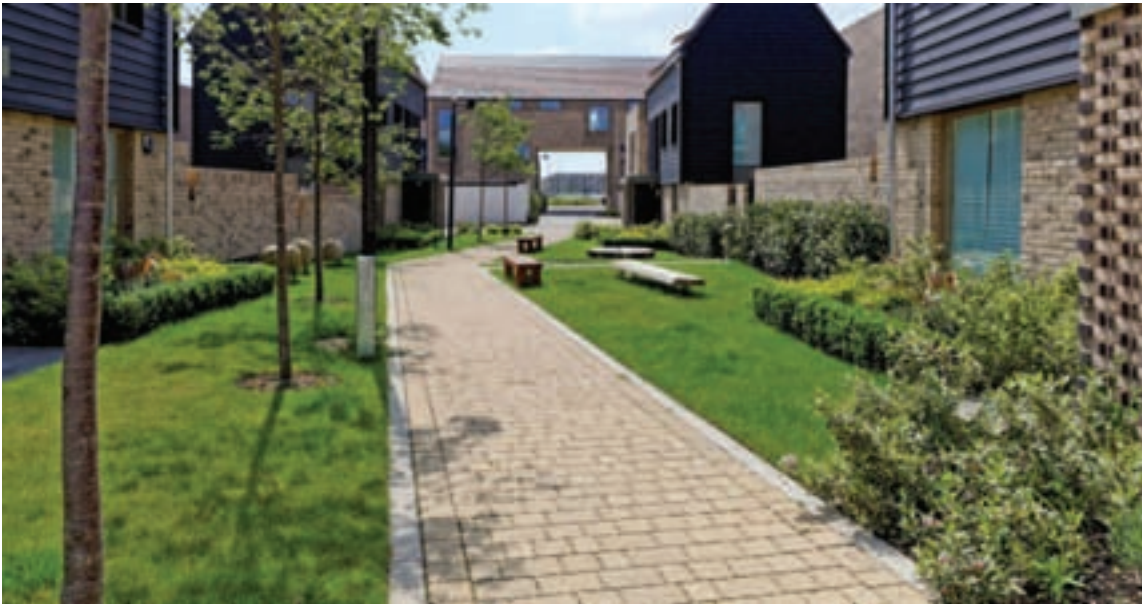
Pictured: Concrete block permeable paving used extensively, with other SuDS techniques, at Proctor & Matthews' Abode housing, Cambridge - Winner of the Housing Design Awards 2014. Photo © Simon Bunn
