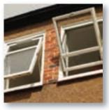
Sheerframe 8000 Top Reversible windows from Synseal fully reverse for ease of cleaning in total safety from inside the building. This specialist Top Reversible window design features a purpose-designed Sheerturn hinge and is ideal for domestic applications including escape windows as well as medium and high rise dwellings and office or hotel accommodation. A range of transoms and mullions provide additional multi-light and stick construction curtain walling
