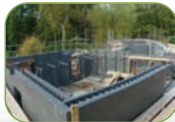
Curved Thermowall Construction.
