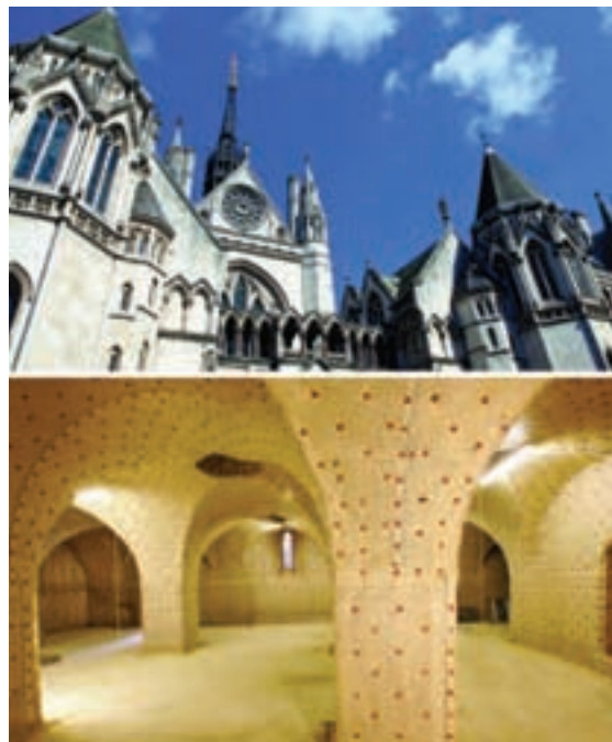
Figure 1: Cavity drain membranes were effectively applied to the interior vaults of the Grade I Listed Royal Courts of Justice, London. Here we can see the completed system, prior to the application of the internal finish
