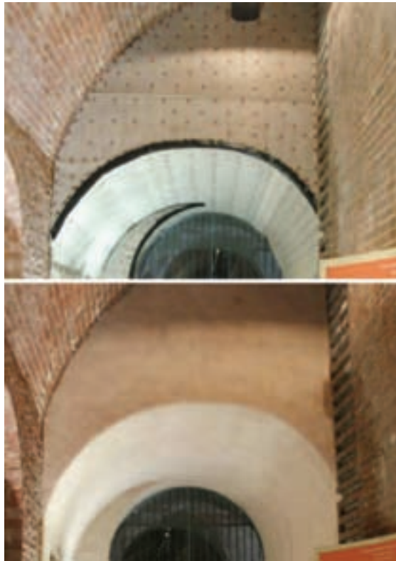
Figure 2: This dry, clean internal wall finish at the Grade I Listed St George's Hall in Liverpool was achieved through the application of meshed damp proofing membranes in order to act as a damp barrier. Here we can see the membrane both pre- and post-application of the internal wall finish
