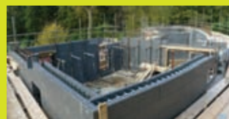
Curved Thermowall Construction
