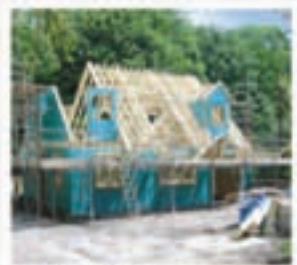
Watertight Frame Erection
