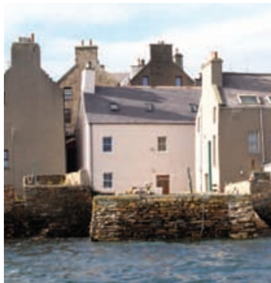
Pictured: A former merchant's house on the seafront in Orkney is a tough test for silicate masonry paint. The owner says sea spray can drive over the house and other paints soon flaked off but, two years on, he remains happy with silicate masonry paint. A bespoke shade was created to match the town's conservation colour palette © Earthborn
