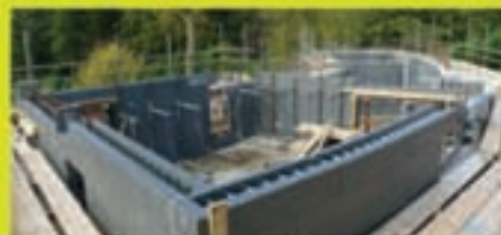
Curved Thermowall Construction
