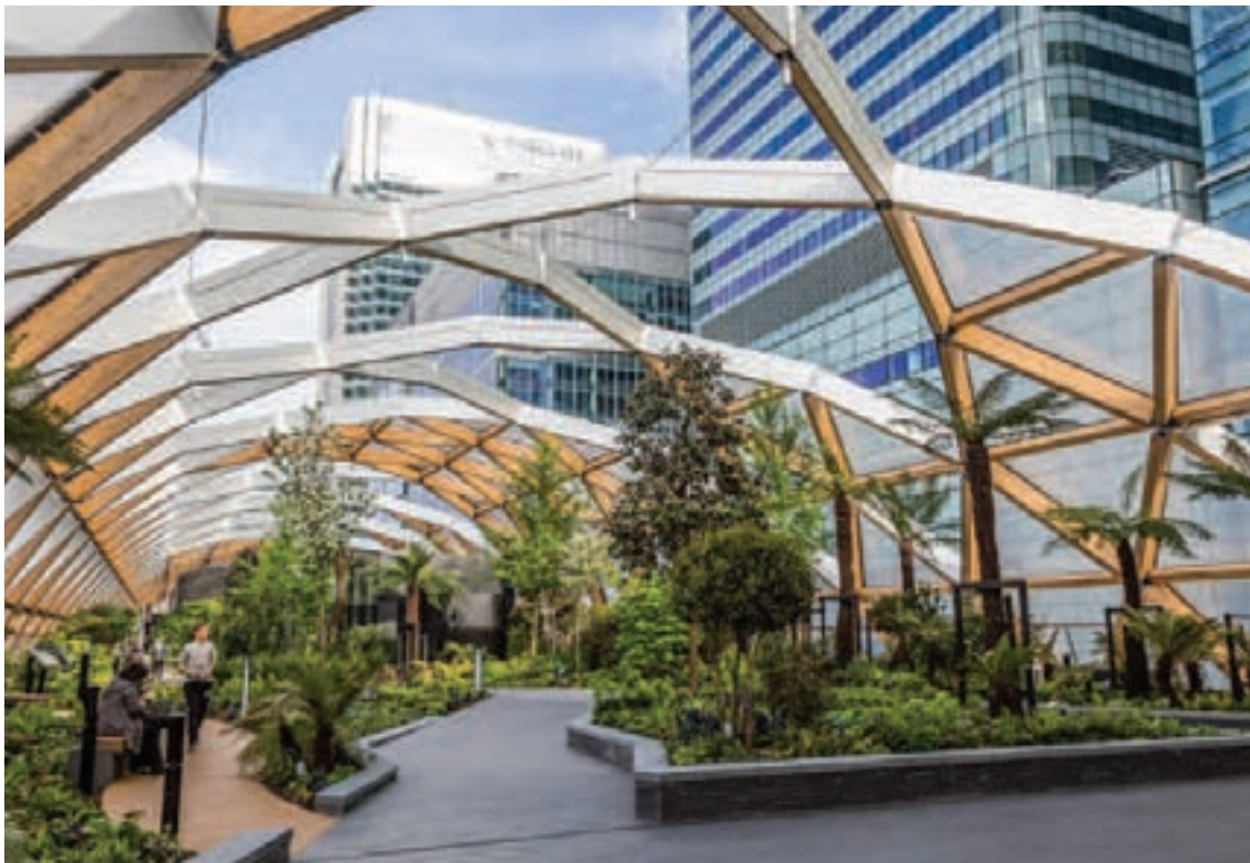
Tropical roof gardens designed by Foster + Partners at Crossrail Place, Canary Wharf with a timber lattice roof and waterproofing by Radmat
