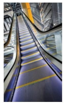
installing an additional stop button on each machine during mid travel. Bespoke manufacture of the machines at 35 degrees instead of the standard NR specification of 30 degrees, and the reduction of the speed of the machines from the standard NR .65m/s to .05m/s all result in safe, efficient travel within the constraints of an unusual and stunning building design. With no room for housing external controllers these became an integral part of the escalators.
