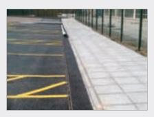
– 100, 200, 300 and 680 because of their overall volume capacities. As well as straight runs of 100 and 200 channels, the 200, 300 and 680 sizes were installed in a step fall arrangement providing an enhanced water volume for these runs of 366,324 litres per metre (l/m). All the sizes supplied had fixed ductile iron, 14mm open slot inlets finished with KTL, a rust resistant coating. All 1229 metres of RECYFIX® HICAP® channel installed complied with loading category
