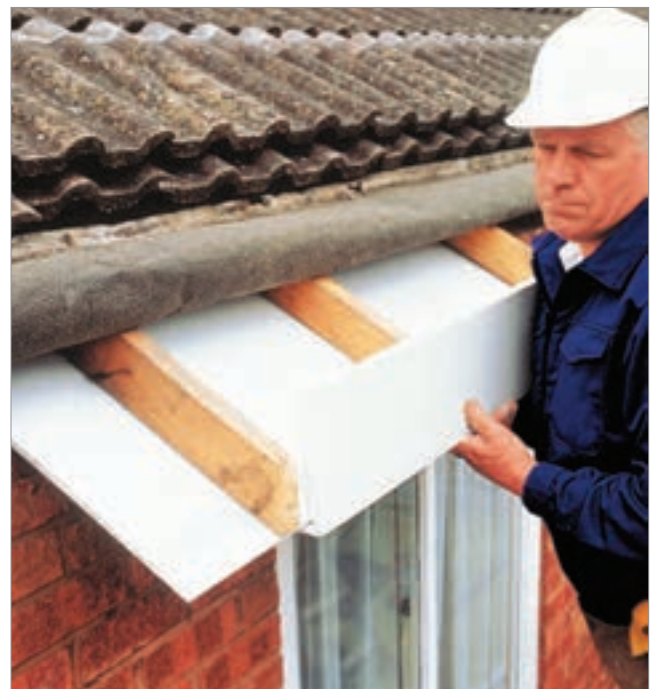
Cellular PVC has similar working characteristics to timber but is far more durable
