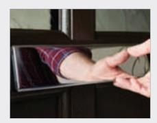
hinge mechanism to prevent attack. The inner flap has a positive stop feature for maximum protection from 'fishing' while the inner flap projection is below door handle height for added protection.
