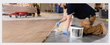
an extremely high initial grab and zero risk of hollow spots. The bond strength of Bona Titan will not diminish over time so the stability of the floor is guaranteed for the long term.
