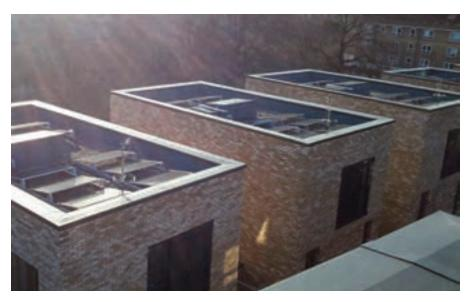
cost-effective way to attenuate storm water flows, by temporarily holding rainwater back on the flat roof. A temporarily retained rainwater depth of just three inches (less weight than a heavy snowfall) on a flat roof would severely reduce ground level flooding and the impact of drainage system overload of even a big storm. The only additional cost to that of a standard flat roof are for slightly higher waterproofing details and a simple flow restriction insert to the roof outlet.
