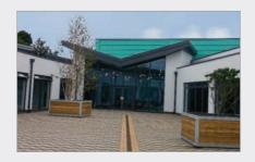
bespoke fascia and soffit with double tiered hoppers. The design further included a butterfly roof and a considerable quantity of wall copings, along with downpipes and more hoppers.
