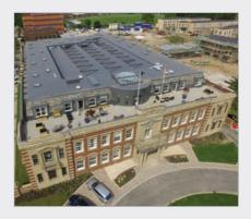
which required zinc on all the vertical faces and Sarnafil on the tops. The flat roof area of the extension was then also covered in the Sarnafil system, along with 140m of parapet guttering detailing, and a new roof terrace area.
