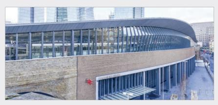
glazing. Each pane of 5.6m glass installed in the lower tier weighed in at 350kg.
