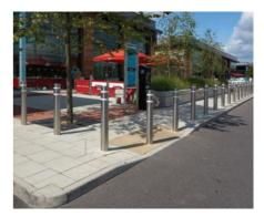
This is a new set of accredited standards that can provide specifiers with access to assured security products designed to stop a vehicle of up to 2.5 tonnes travelling between 10 and 20 mph
