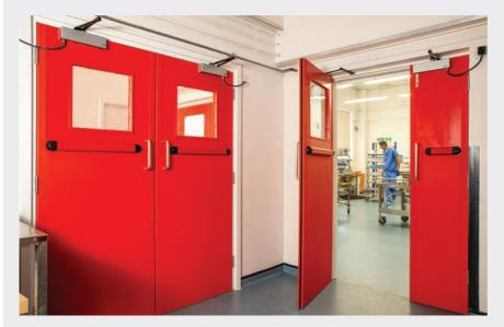
door protection products were used to refurbish and then protect from further impact damage. Door edge protectors were fitted to the leading and meeting edges of the doors with door protection panels installed to a height that would shield the most vulnerable areas.
