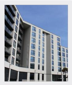
system. The seaside location also meant the windows required a low solar gain and the 0.28 G-value of the 2500 window ensured that the building would not overheat.
