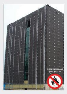
New Powerlon FlameOut Breathe Class A breather membrane is rated Euroclass A2-s1,d0, the highest level of fire protection for wall and roof installations
