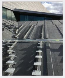
individual supports and more than 3,600 individual bolt heads securing the steel to the slab.
