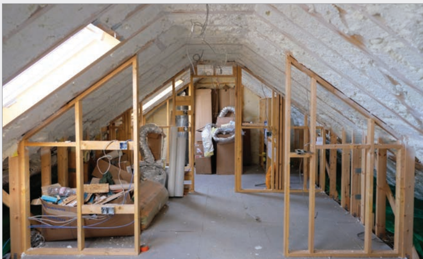
Open cell foams such as Icynene FoamLite are vapour open and allowing the building to breathe naturally.
