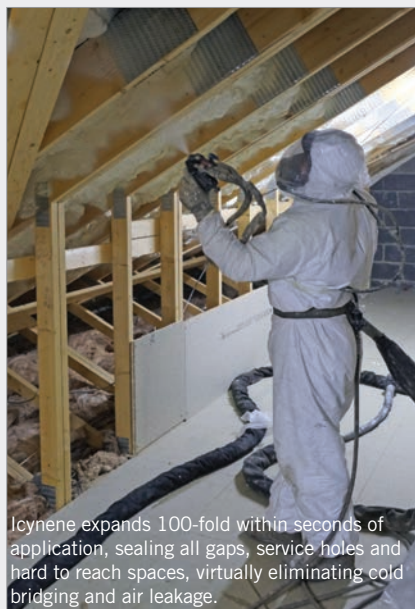
This new generation of spray applied insulation products can result in near zero air leakage through the building envelope.
