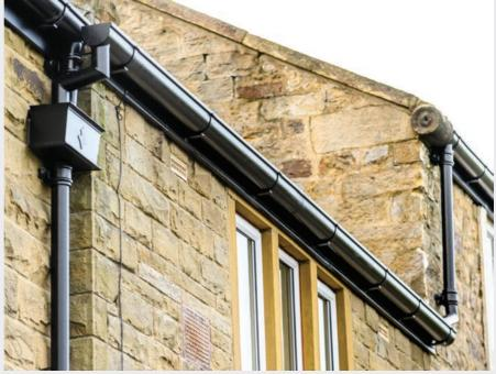
included the replacement of the old discoloured and worn PVC gutters and downpipes along with the rotting timber fascia.
