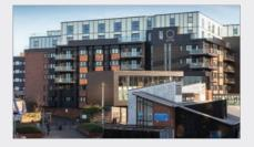
Working in partnership with the Globe Consultants, Ash & Lacy proposed the use of its exclusive MechSlip facade. Developed in conjunction with Ibstock Kevington, MechSlip is a lightweight, mechanically fixed system that offers significant advantages including reduced installation times and associated costs, as well as being completely non-combustible.
