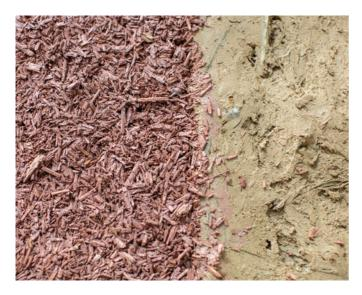
A close up of the thermal (left) and structural elements of a CobBauge wall
