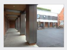
large surface areas of the column casings. Also, the pattern helps provide some additional rigidity to the aluminium, making it even more durable and ideal for high traffic use. The same applies to the ceiling soffits and fascia, but the main advantage of using the same material is the it integrates with the column casings and provides a uniform finish to this excellent project."
