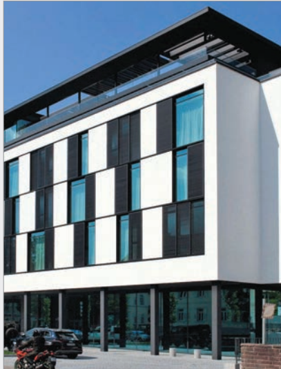
The risk of thermal bridging is at the points where the cantilever steel roof girders connect
