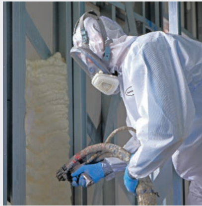
Icynene foam insulation is one of the most effective ways to reduce heat-loss from buildings
