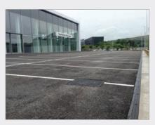
iron HEELSAFE 6mm slot grating to loading Class D400 were installed at the new VW Group dealership at The Point, Llandudno Junction, Wales.
