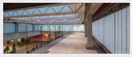
protection, maintaining privacy for the residents and controlling light pollution, while bathing the interior with diffused daylighting, regardless of the weather. The panels are lightweight but very durable with excellent resistance to impact and scratching. They are also vandal resistant with good protection against windborne debris.
