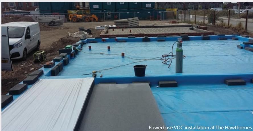
Powerbase VOC installation at The Hawthornes
