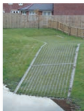
Grasscrete; water attenuation including SUDS
