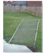
Grasscrete; water attenuation including SUDS
