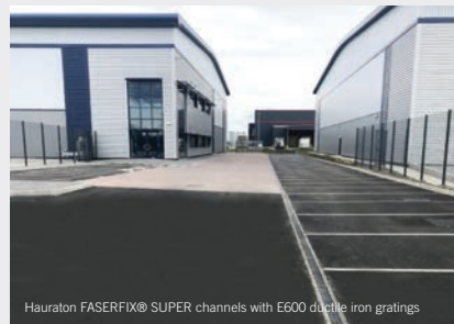
Hauraton FASERFIX® SUPER channels with E600 ductile iron gratings
