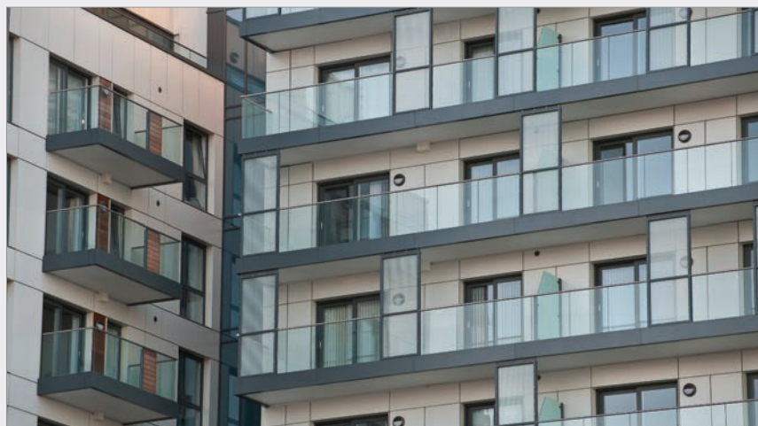
TAPER-LOC® frameless glass balustrade system from CRL can be installed from the 'safe-side' of the balustrade, avoiding the need for time-consuming and expensive scaffolding
