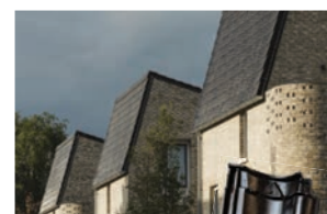
Crest Nelskamp specifically designed 70° angle H14 black clay roofing tile. The unique roofing system flows without interruption continuously from eave to ridge.
