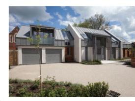
Resin-bound paving is known for its ability to allow water to pass through the material, making it SuDS-friendly and puddle-free
