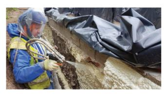
Icynene insulation is applied as a two-component mixture that comes together at the tip of a gun forming a foam that expands within seconds of application
