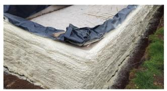
Icynene forms a moisture and airtight seal around the complex network of heating and filtration components and brings the pool up to modern standards
