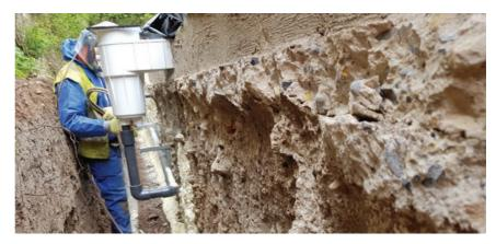
When the pool was built, no external formwork had been used so the wall faces were rough and uneven
