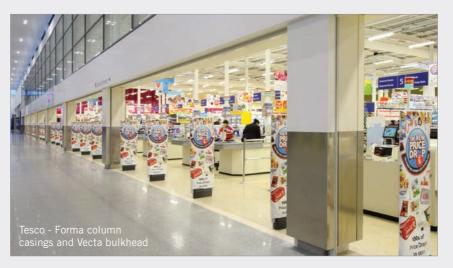
hours fire protection. Originally designed for mezzanine support columns, Metza is also used in food retail fitted with corner protectors to resist scuffing and damage caused by shopping trolleys.
