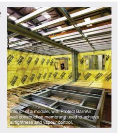
to help us meet the detailed specification, using materials that we know are tried and trusted. In particular, the use of BarriAir helped to achieve strict airtightness and vapour control, contributing to an outstanding energy efficiency rating for both properties that exceeded Building Regulation requirements. Protect understood our needs and provided detailed technical support along the way, whilst ensuring our products were delivered on time to meet our busy schedule."
