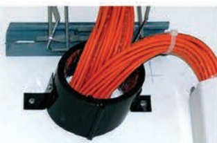
COLLARS CAN BE USED FOR PIPES AND ALSO CABLES
