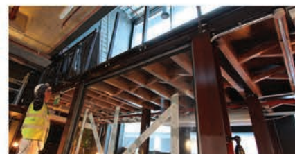
Product 83 - Intumescent coating for steel for upto 90 minutes protection to structural steel.
