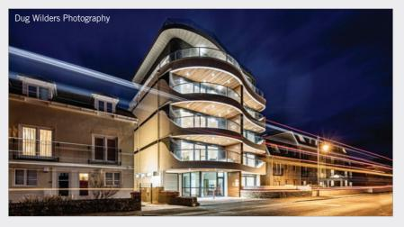
large sea-facing balconies with generous curves. The detailing of these balconies is critical though, if thermal bridging is to be minimised and the energy performance not compromised.
