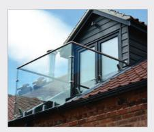
"We were quickly able to visit the site, advise the client on the best course of action, and deliver a complete solution in a very short period – supplying 25m of stainless steel tube and 30 square metres of toughened laminated glass alongside the spigots, stiffeners and fixings."
