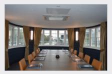
The Series 20 vertical sliding units were faceted onto the curved on plan original bay windows on the ground and first floors. This was to provide adequate thermal and noise insulation to the restaurant and meeting room. The Function room was fitted with the Series 15 3-pane horizontal slider, which can support thicker glass when higher levels of noise insulation are needed.
