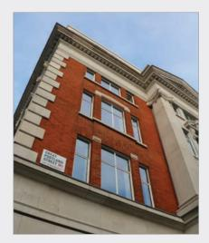
glass units featuring solar control glass to the outer pane. Black framed ground floor windows were also supplied by Crittall.
