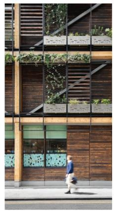
of this strongly expressed diagonal structure, and the cantilevers, which echo other Sheppard Robson buildings in the area (3 Hardman Street, and 1, the Avenue, which is tenanted by Armani, and has a 27 metre cantilever). Allen-Burt says that in designing an exposed external structure, it's important to "work very closely" with the structural engineers (in this case Engenuiti), otherwise the facade can "become a structural solution rather than an architectural one."
