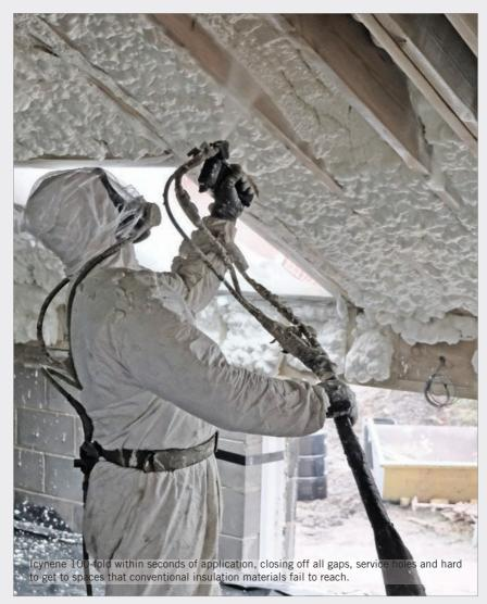
open cell material with a soft, yielding texture. This not only provides outstanding insulation properties, but also allows the building to breath naturally, resisting internal condensation – particularly important when insulating older, heritage-type buildings.
