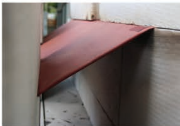
SEALED CAVITY TRAY
