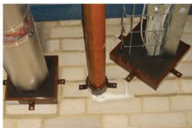
DIFFERENT SERVICES FITTED THROUGH COLLARS AND MULTI PURPOSE BOXES
