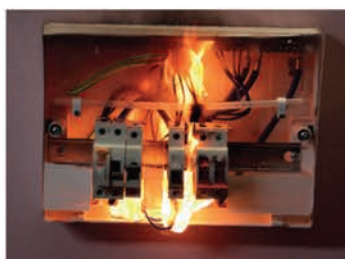
ENVIROBURST - FIRE IN THE CONSUMER UNIT BEFORE BURSTING
