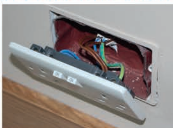
ACOUSTIC & FIRE GASKETS FOR DRY LINING BOXES
