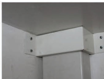
INTUMESCENT SADDLES FOR PIPES AND TRUNKING
