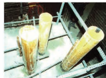
FIRE AND INSULATION PIPE IN CONCRETE CEILING. 4 HOUR PROTECTION
