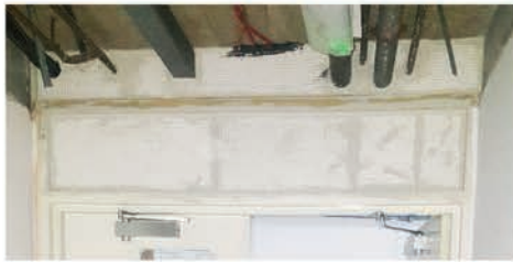
SEALING SERVICES THROUGH WALLS
