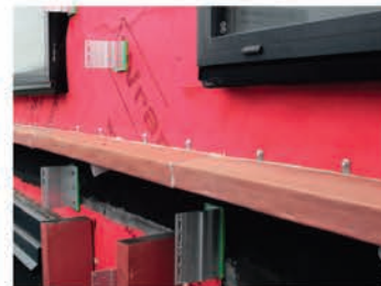
RSM - CAVITY BARRIER FOR RAINSCREEN FACADE SYSTEMS
