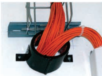
COLLARS CAN BE USED FOR PIPES AND ALSO CABLES
