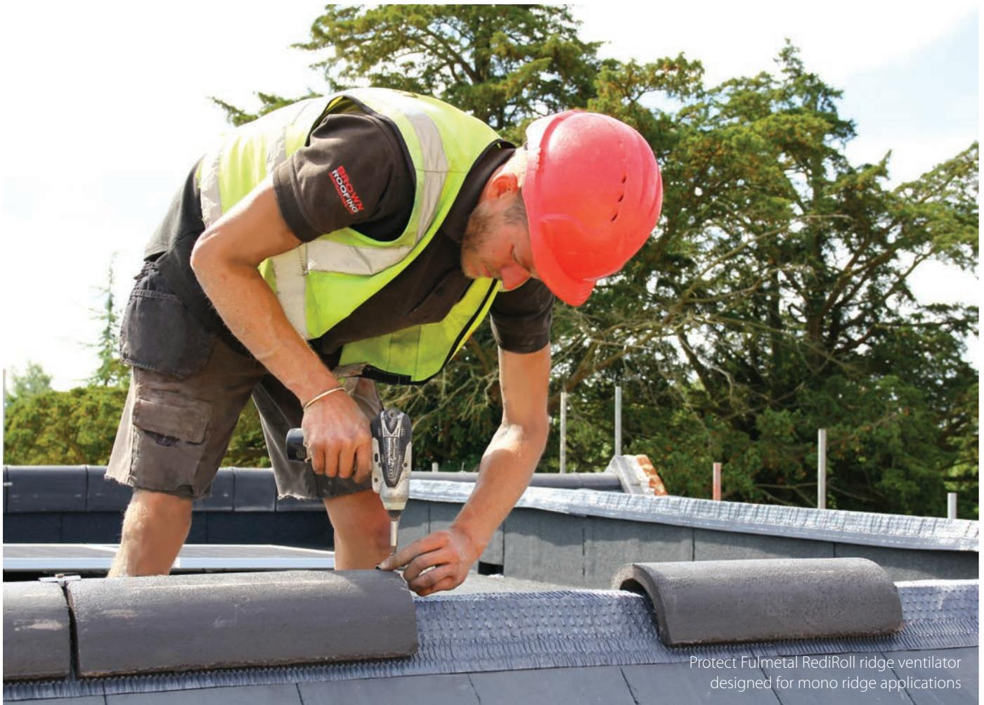
Protect Fulmetal RediRoll ridge ventilator designed for mono ridge applications
