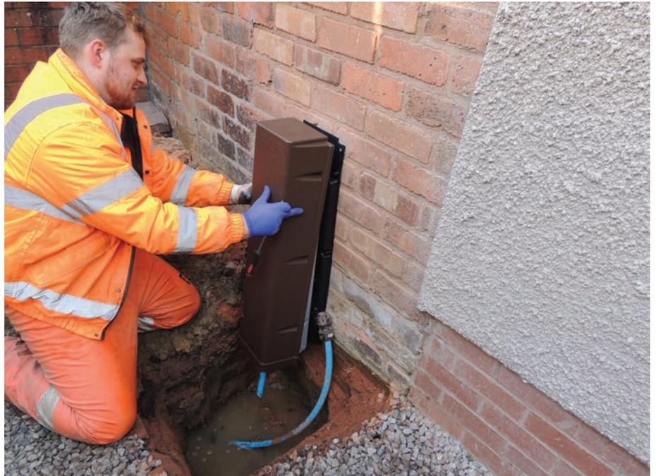
to be installed, as it is designed to provide frost protection for up to three 32mm OD water pipes installed to the exterior of the building.
