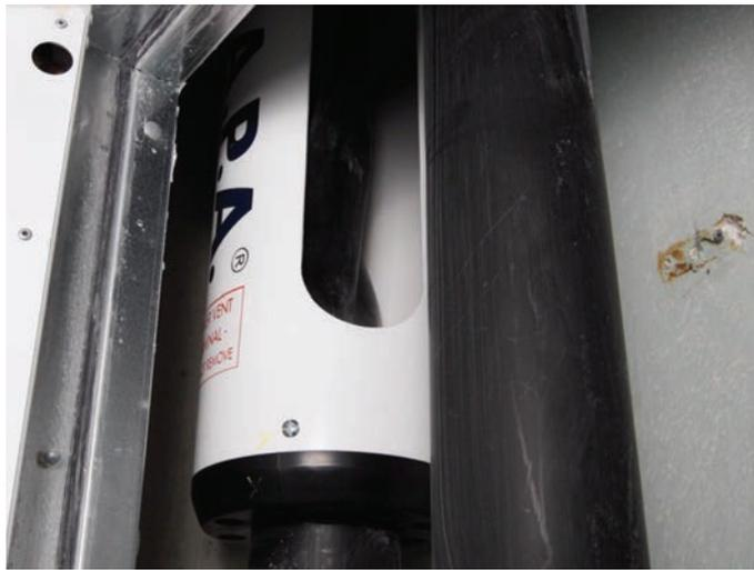
A Positive Air Pressure Attenuation system with an air admittance valve provides a drainage ventilation system that helps control nuisance air pressure regimes which otherwise would establish themselves within the soil and waste system as water building, often from great heights
