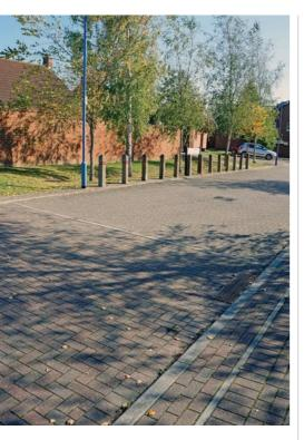
provide a completely level, well-drained, firm and slip-resistance surface accessible to all, without the need for cross-falls, channels, gulleys or other interruptions. These and other savings resulting from SuDS are being demonstrated at the Lamb Drove SuDS Monitoring project in Cambridgeshire.
