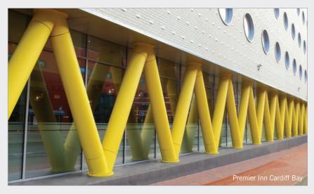
solution. Forma, in particular, provides specifiers with an exceptional scope of options and can be specified in a range of shapes including circular, up to 1000 mm diameter, or as square, rectangular, hexagonal or bespoke forms.
