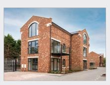
heavy-duty brick slip feature arch lintels for ground, first and second floor openings with a 1085 mm span and 543 mm rise. Over 40 brick slip arches were manufactured by Keystone's production team to a high quality and consistent finish. Each Hoskins Maltings Antique brick was cut to size and bonded using a BBA-approved construction adhesive to the load bearing lintels. The patented perforated lintel design of a Keystone Brick Slip Feature Lintel allowed the adhesive to
